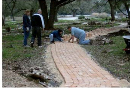
Laying the pavers for the walks.
